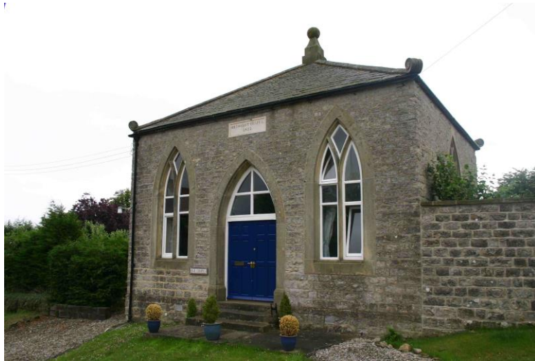
Fig 5. Former Methodist chapel, Edstone (2010)
