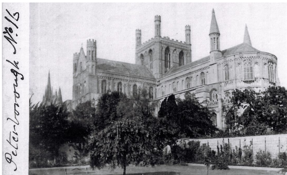
Photograph showing three of the Dean's 'chimneys'
