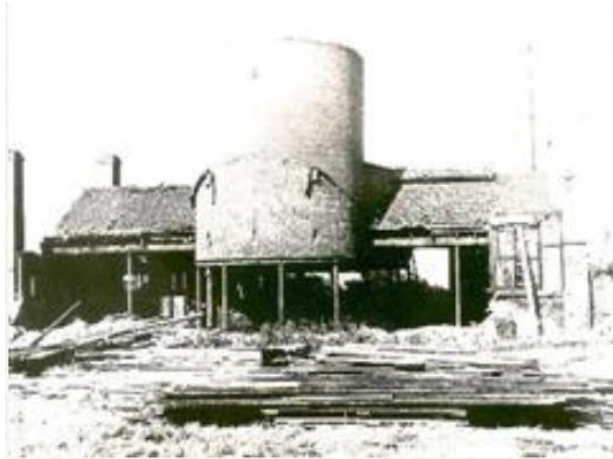
Chemical Works before demolition (photo Archive 1858 - (seahamfamilyhistorygroup.org.uk) )
